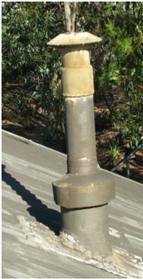
The Flue (Nest at roof level)
